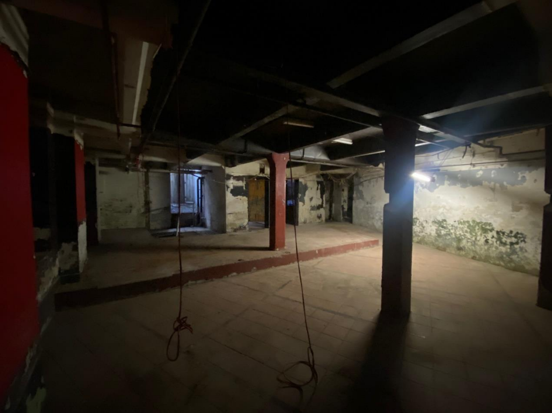
Figure 7: Interior, basement level
