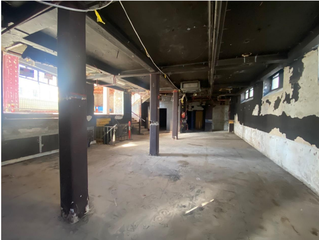
Figure 8: Interior, lower ground level (basement)
