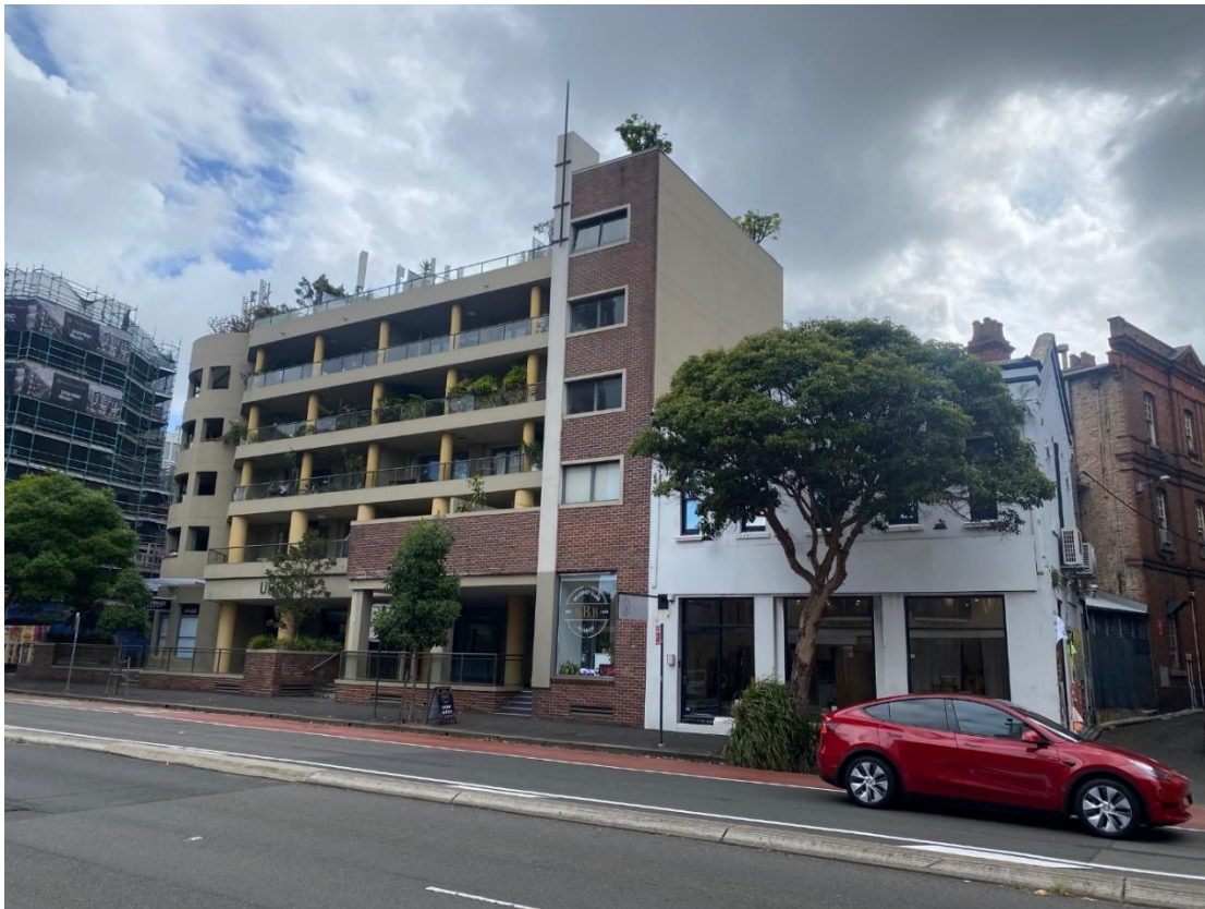
Figure 17: Development on opposite side of Patterson Ln (Flinders St frontage), looking southeast
