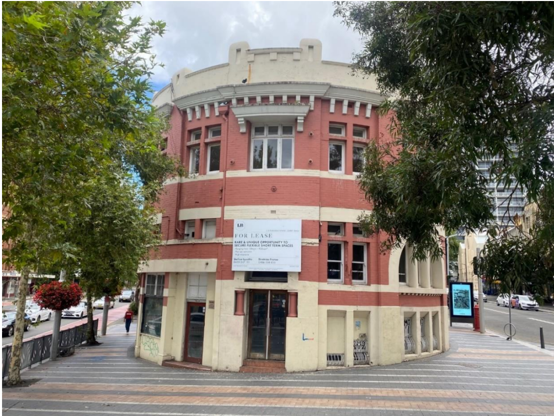
Figure 2: Site viewed from Taylor Square, looking south
