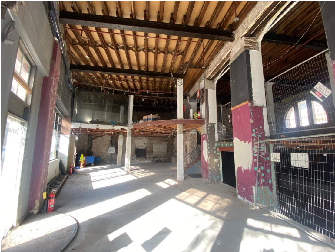
Figure 9: Interior, ground floor level
