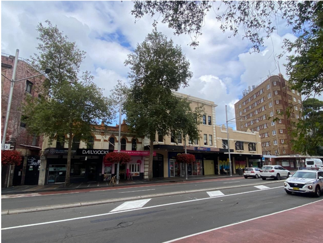
Figure 18: Development located on the opposite side of Flinders Street, looking east
