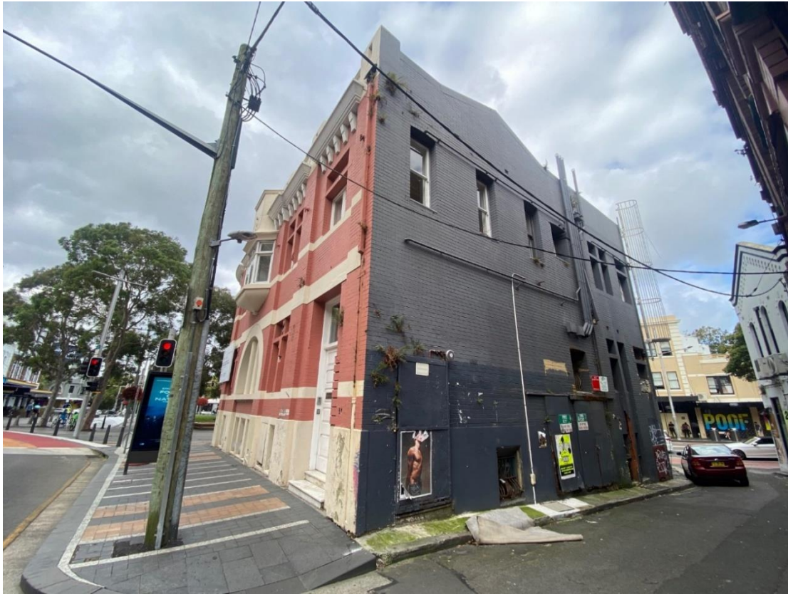
Figure 4: Site viewed from the opposite side of Patterson Lane, looking north east
