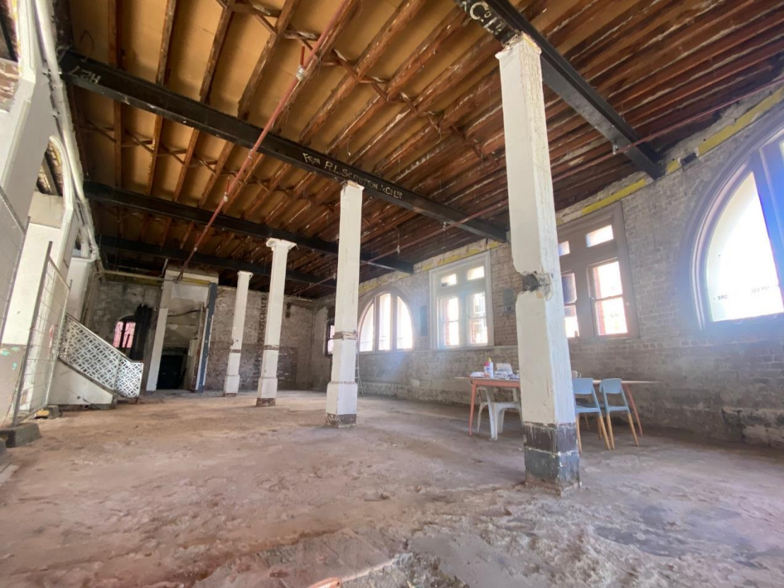
Figure 10: Interior, upper ground floor level
